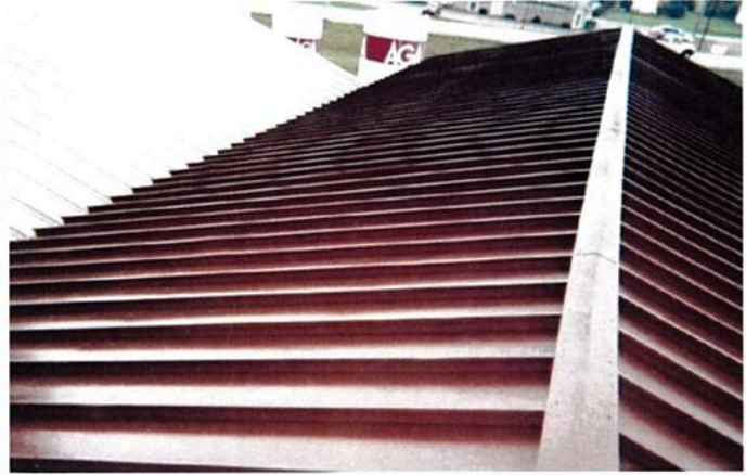
FINDING A FIX A project for Linde Gas in West Virginia required application of Elastomeric coating to revive an existing metal roof.
