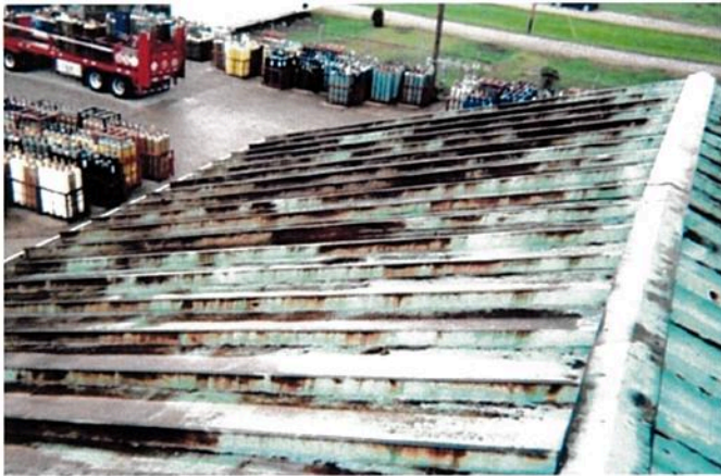
FINDING A FIX A project for Linde Gas in West Virginia required application of Elastomeric coating to revive an existing metal roof.
